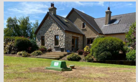
▶ Retrofit of Tricel Vitae plant
