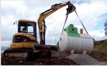
▶ Tricel Vitae 6 being installed
