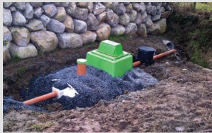
▶ Tricel Vitae 6 installed
